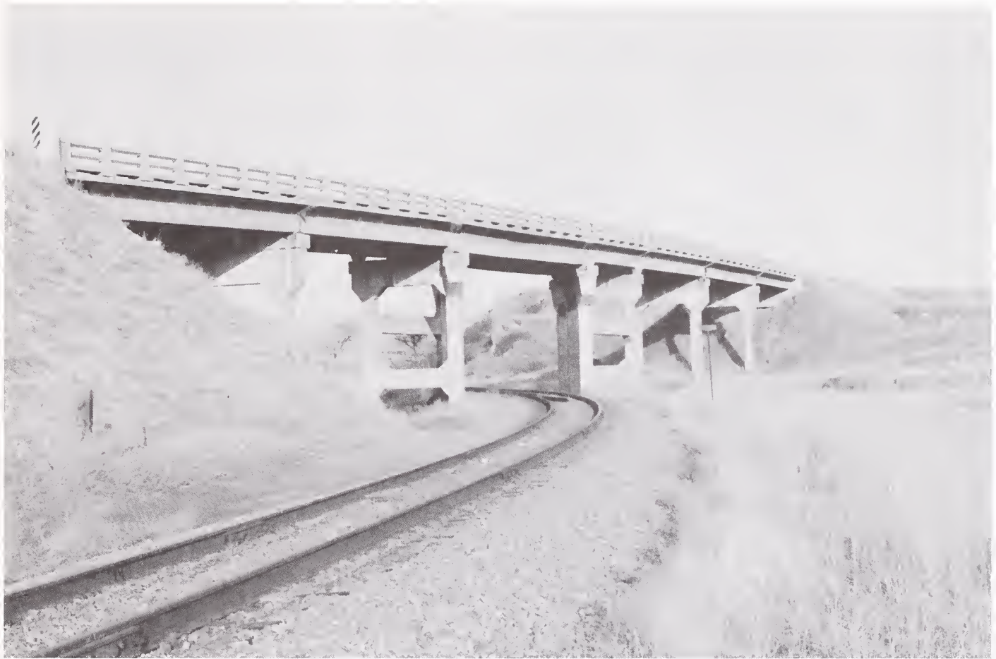
Northern Pacific Overpass, built in 1934.
